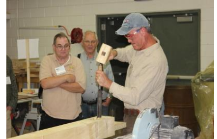
John Pflug using a 1" X 1" 90° Mortising Corner Chisel to Square-up the inside corners of the mortise.
