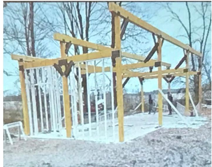
John Phlug showed off some photos of a timber frame structure that he was building. All of the tenons and surface pockets were cut by CNC so that the structure would fit together like a puzzle. Um...yeah. Wow. Very impressive John!
